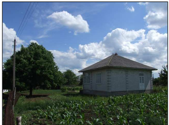
The property before remodeling began for the church in Terebna, Moldova.
